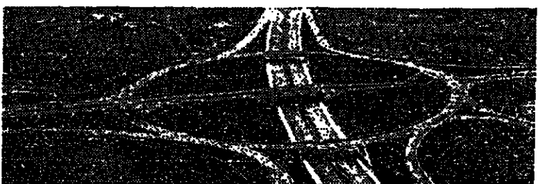
M42 Birmingham - Nottingham Motorway (Solihull Section) for Midland Road Construction Unit, Department of Transport Interchange with the A45 Birmingham Coventry Road. Main Contractor: R. M. Douglas Construction Limited. Surfacing by: R. M. Douglas Asphalt & Paving Limited
